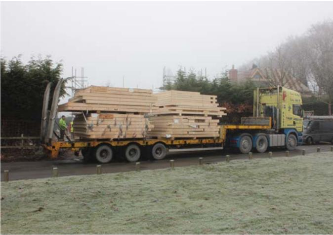
The team arrive on a cold Monday morning, three weeks before Christmas. The sub zero temperatures and driving rain would normally have put a stop to most construction projects, but the panelized nature of SIP's means they can be installed in almost any conditions.
