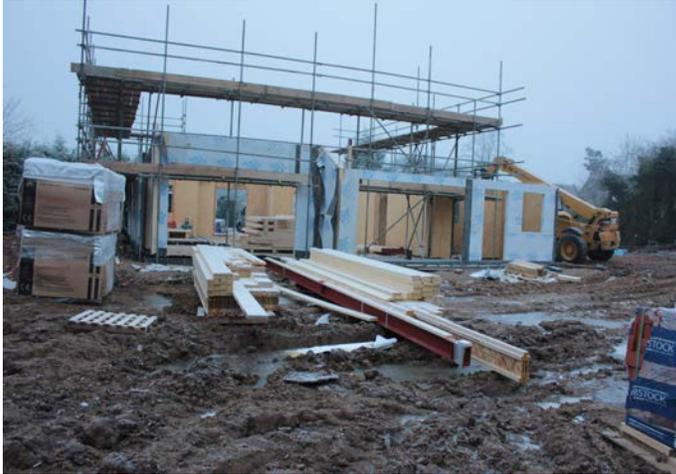
Once the walls were upright and sealed together the team could install the joists that would become the second floor of the house.
